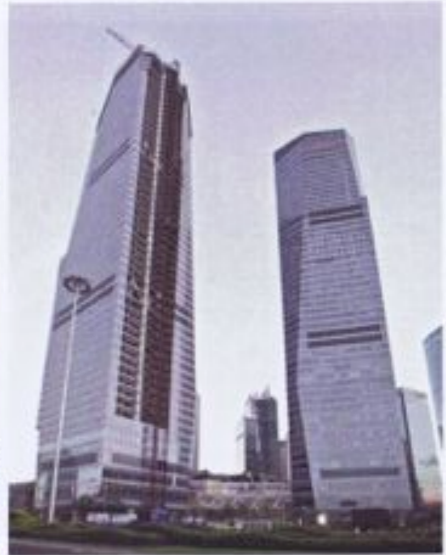
Shanghai IFC North Tower, 2010
