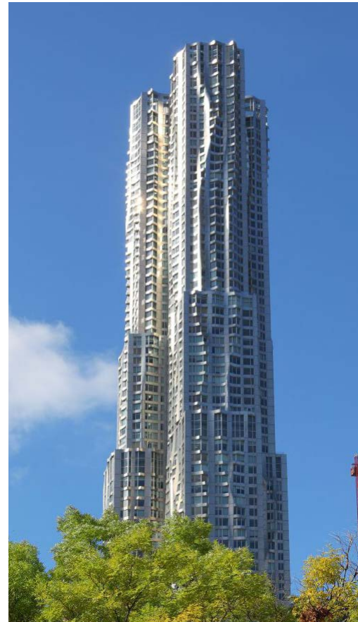
8 Spruce Street, New York, USA
