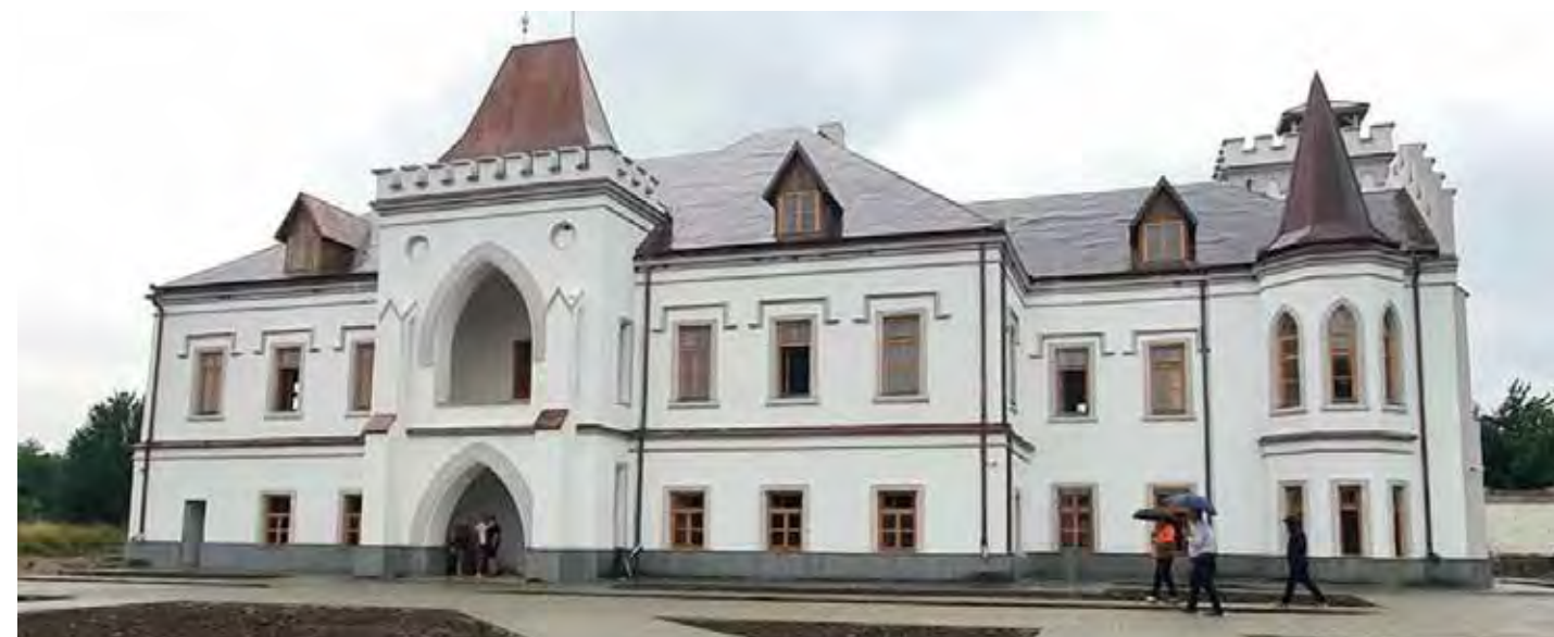
Restaurare castel NOPCSA, sat Săcel, jud. Hunedoara, acces principal
